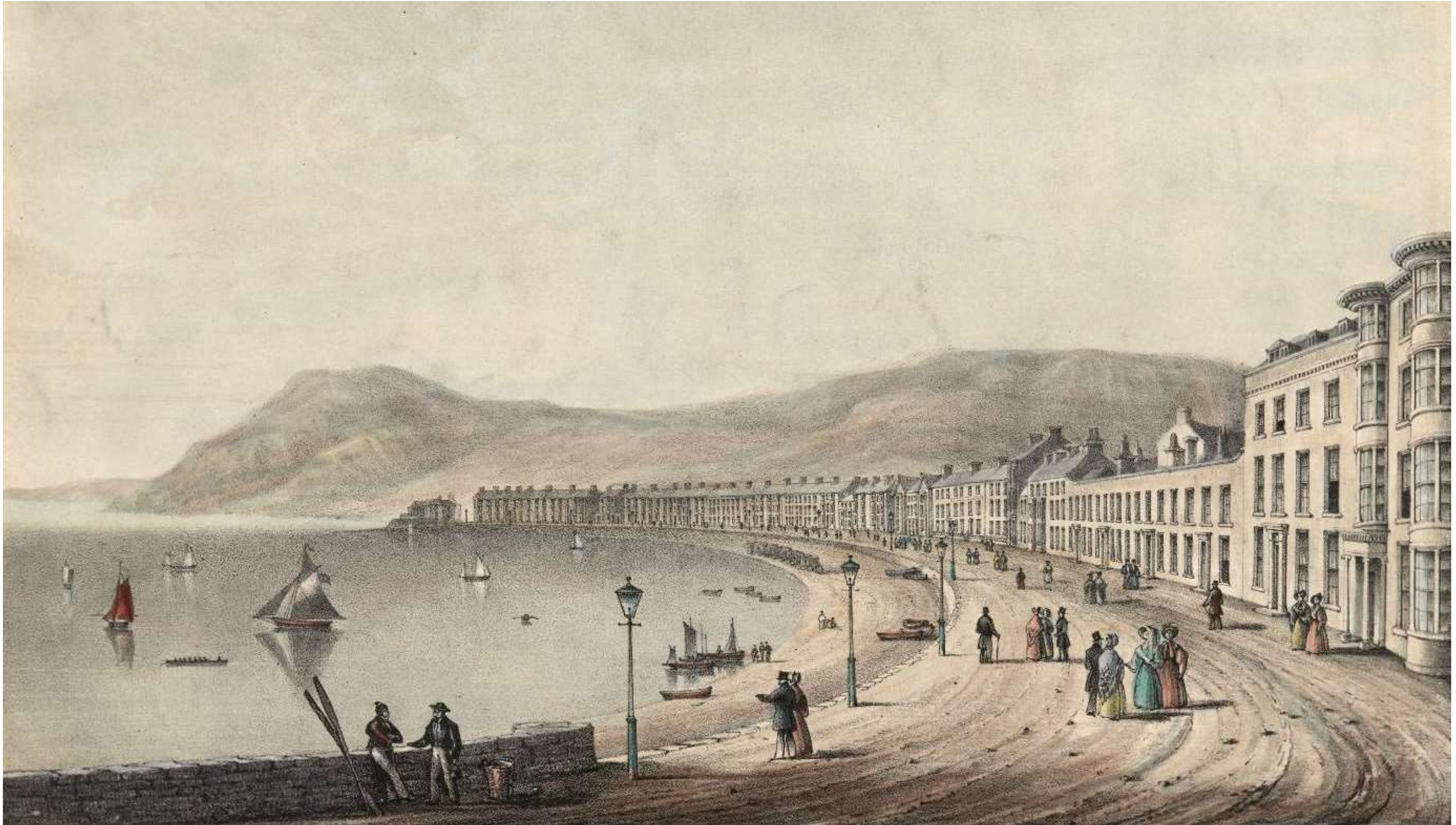
Marine Terrace, Aberystwyth, William Crane circa 1840 (Wikimedia Commons). Most of the properties at this period conform to a set of standards that give it visual coherence - three storey buildings with small pane sash windows. Bow windows were popular in the early 19th century prior to the council's imposition of canted bay windows as a preferred standard. The Belle Vue Royal Hotel can be seen in the middle ground to the right hand side of the Ty Belgrave gables. There are no dormers in this early view.
