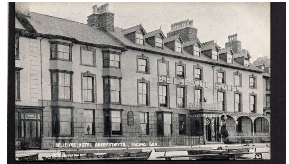
Late 19th century. Top: The left hand block has full height bay windows common in Aberystwyth from the second half of the 19th century. Bottom: Image shows the gabled cross range to the far right, with its own porch, bay windows have not yet been added.
