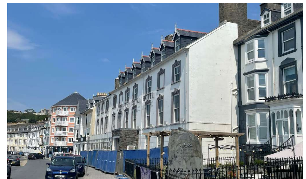
The rear and front setting of the Belle Vue Royal Hotel. The front elevation has been hoarded since the 2018 fire, and the gabled cross wing to the north demolished.
