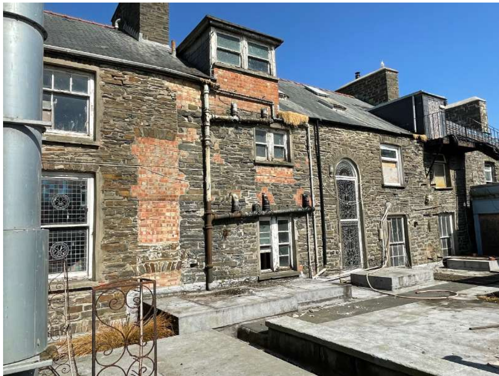
Main Block rear elevation at ground and high level
