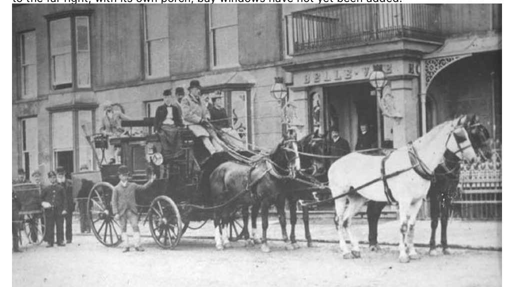
Belle Vue Royal Hotel circa 1890s. The vertical glazing bars to the sash windows have been removed in favour of large panes, and the portico railings have been simplified
