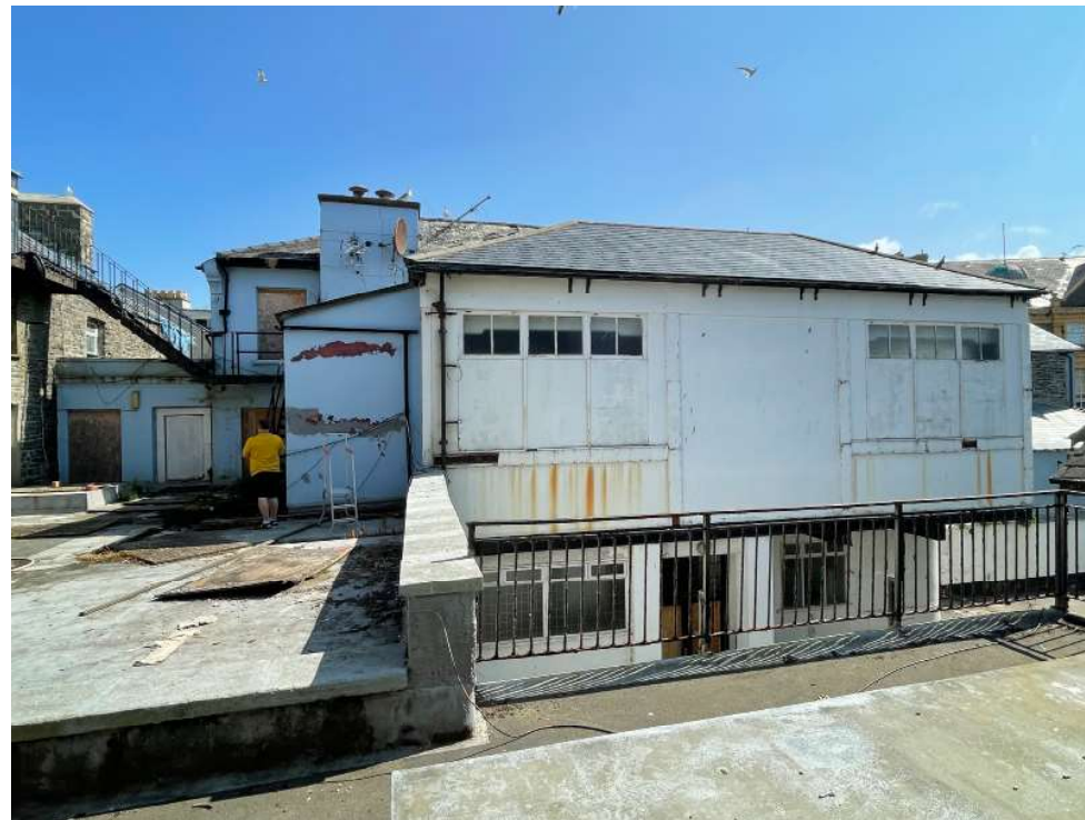
Ballroom Wing south elevation at ground and high level
